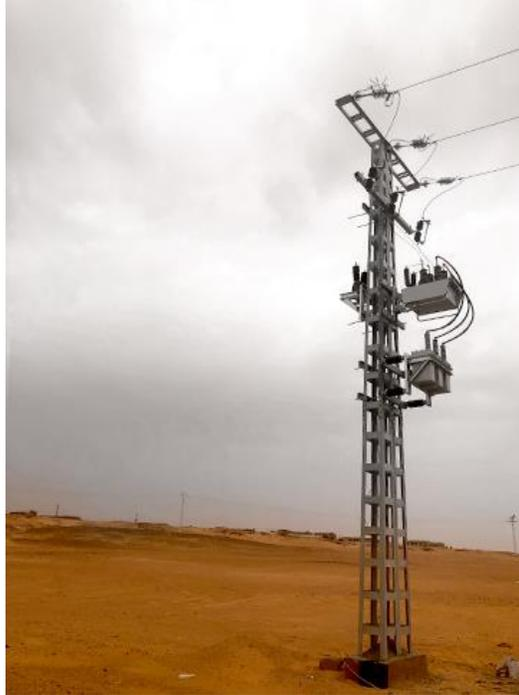
*Pole Mounted Capacitor bank switching,*
