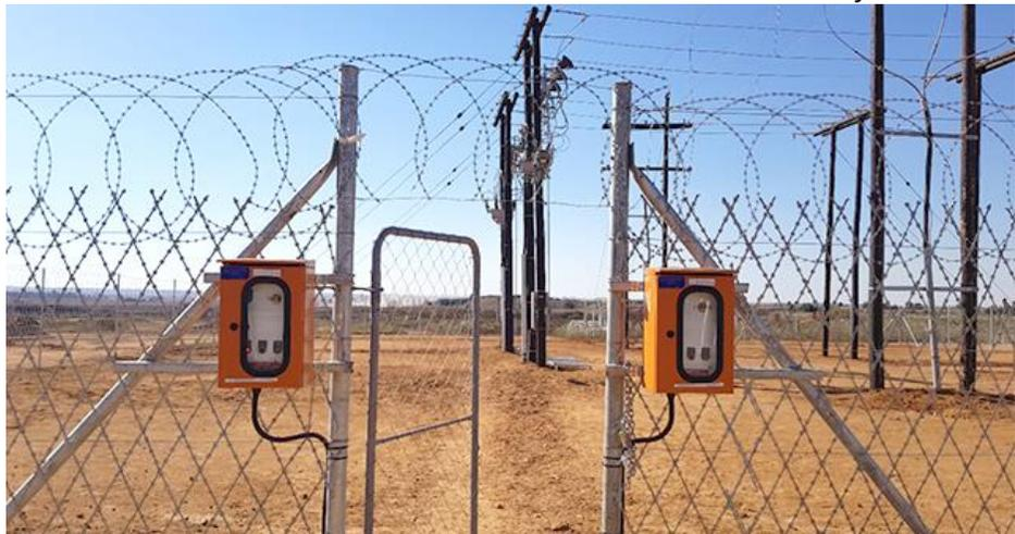
*Interlocks connected to the OSM Reclosers in the Switch Yard*
